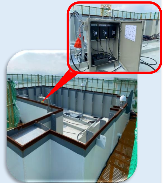
<Top of the bridge>
